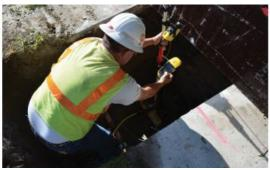
It used to take Questar Gas inspectors half an hour to collect pipeline assets on a site and then eight weeks to produce a final map of the work. Today, using GNSS technology, data collection takes 10 minutes and the map is available instantly, reports Vivienne Wallace.
