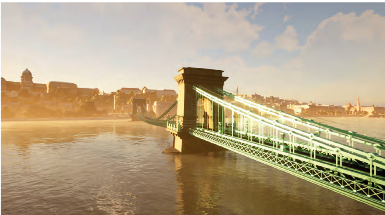
▲ The Széchenyi Chain Bridge in Budapest is facing complicated restoration work.
