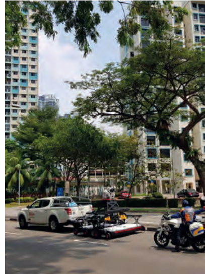
◀ Figure 4: Exploring the use of ground penetrating radar in mapping subsurface utilities.
