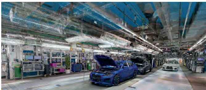
▲ As part of the collaboration, NavVis IVION will connect to NVIDIA Omniverse, allowing users to stream reality-capture data for factories into Omniverse simulations via the USD framework. (Image courtesy: NavVis)
