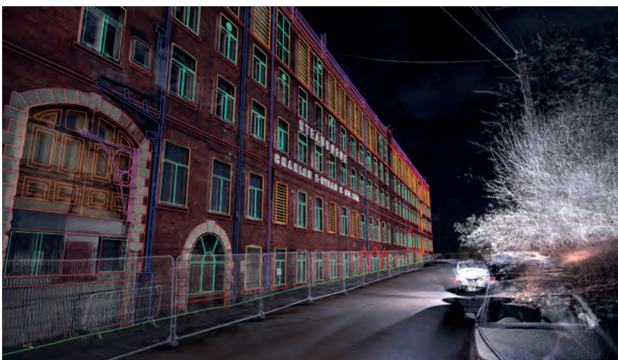
▲ A commercial building facade, Leeds.
