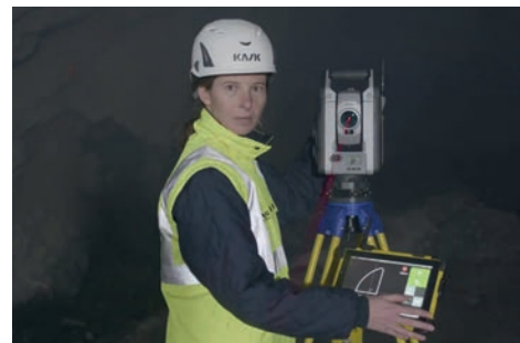
▲ The collaboration provides a full-featured workflow specifically for tunnel construction surveys.
